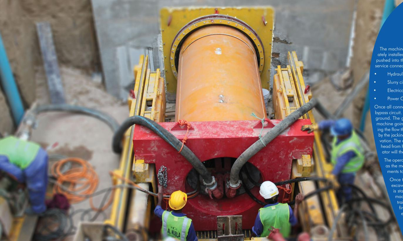
The machine is powered hydraulically. The source of this hydraulic power is a power pack situated in the can immediately installed after the machine. Initially the machine is lowered onto the jacking frame and the cutter head carefully pushed into the shaft seal using the jacking frames hydraulic jacks. Once in position all the services are connected, the service connections consist of
